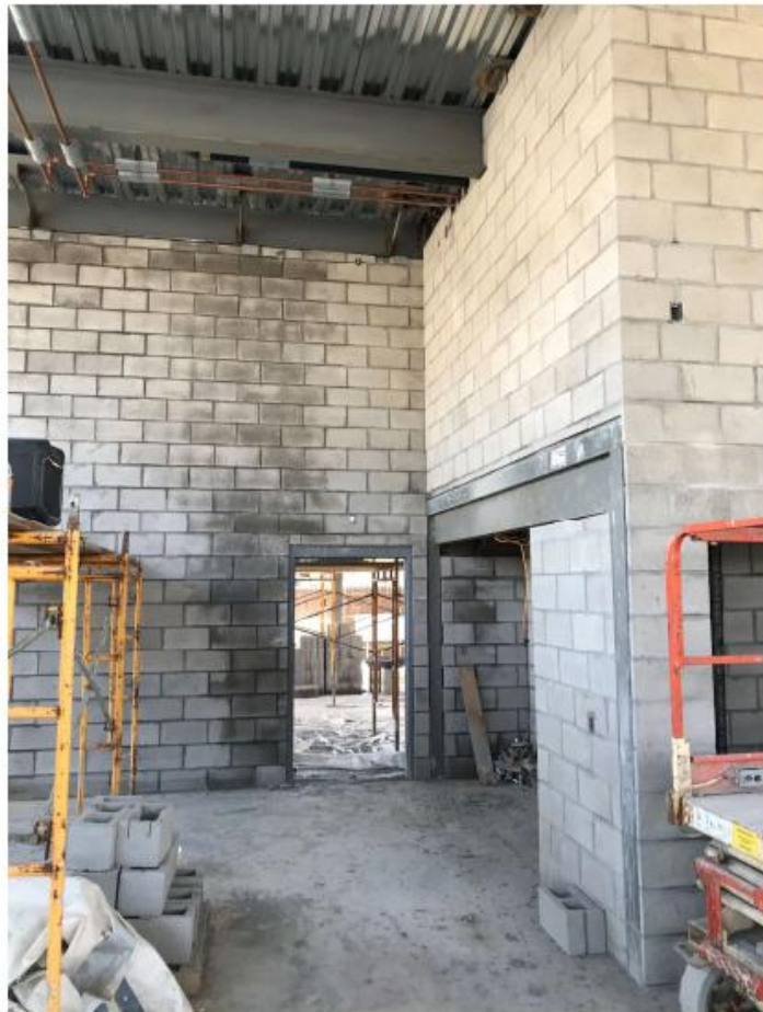
Photo 2: Installation of the interior CMU non-shear walls.
