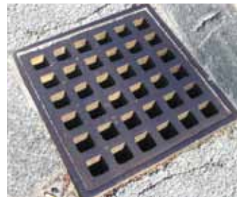
Stormwater enters the storm drain through this catch basin grate.
