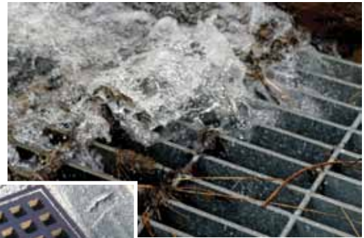
Stormwater enters the storm drain through this catch basin grate.
